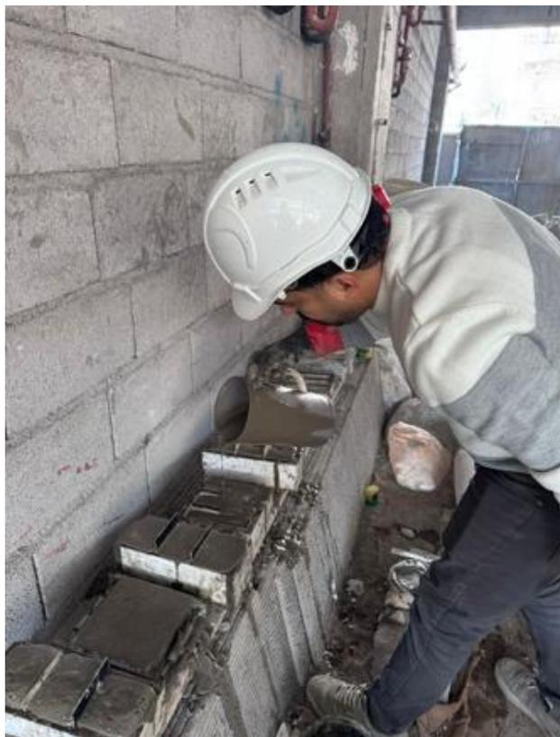
Figure 1. Pouring the FC into molds.
